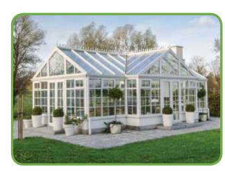
All Vertex roof options have a unique one piece GRP peripheral main beam that incorporates an integral gutter, giving the roof much greater inherent strength. The ring beam is available with or without dentil moulding. The design is fully flexible, with options available for Victorian, Edwardian and P shaped designs, so you can create a style that suits your home.
